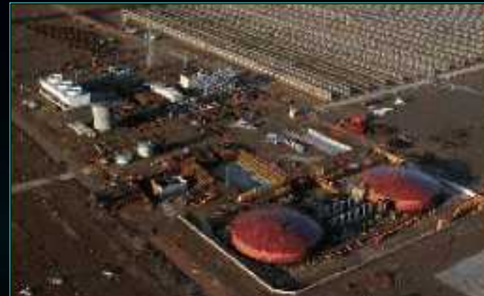
Under construction near Grenada, Spain 50 MW plus 6 hours storage
